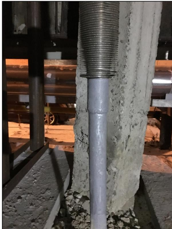
**Figure 5:** Thermosyphon near Pile
