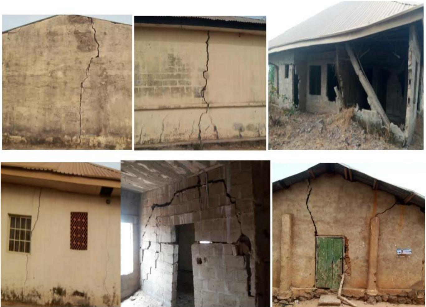
**Figure 3:** Vertical and diagonal Cracks on buildings
