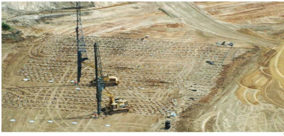
Figure 2: Geocomplex vertical drains are placed in the ground by using a special crane with a vertical guide, in close in-between distances of 2-4 m (Source: Kaltsios 2012) [3].
