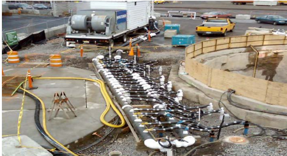
Figure 6: Soil cooling layout for stabilization. (Source: Platis-Vigenopoulou 2016) [7].
