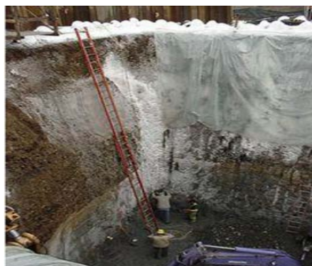
Figure 7: Application of the cooling method in a deep excavation. (Source: Platis-Vgenopoulou 2016) [7].
