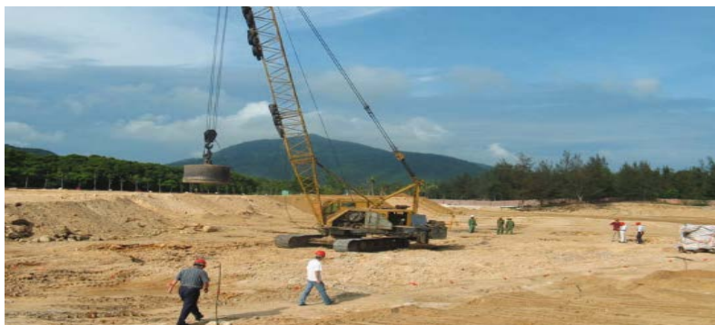
Figure 1: Application of the dynamic compaction method, which consists of dropping large weights onto the ground. (Source: Kaltsios 2012) [3]
