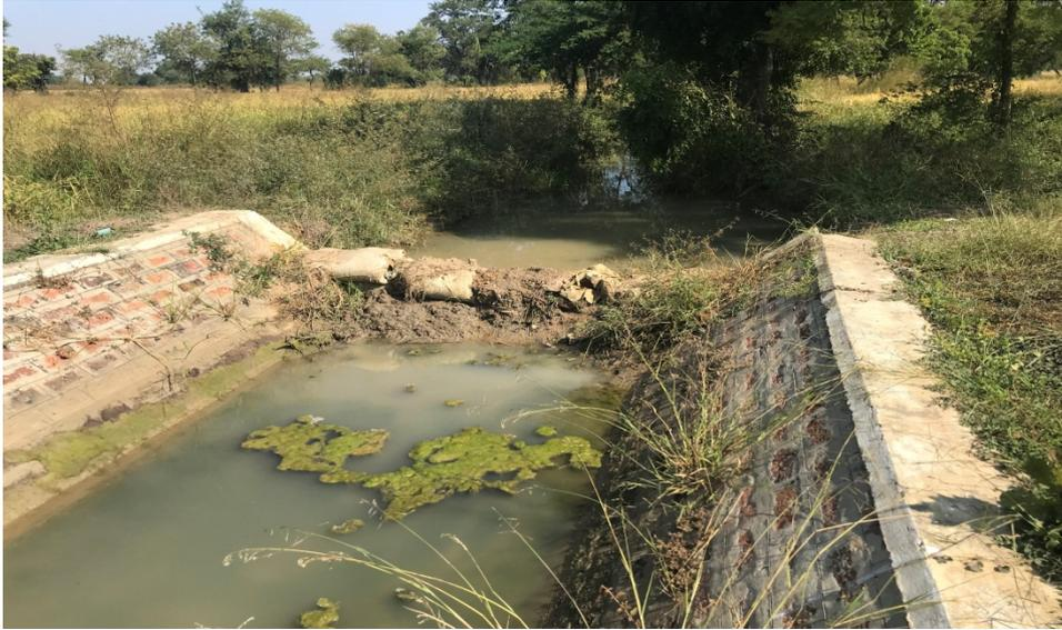
**Figure 5:** Illegal conveyance means with use of sand bags and wood logs in Kyan Kin Village
