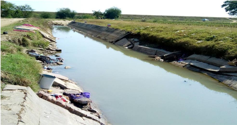
**Figure 3:** Deterioration of canal Lining in Kyaukthanbet Canal, Mattaya Township, Saedawgyi Irrigated Area
