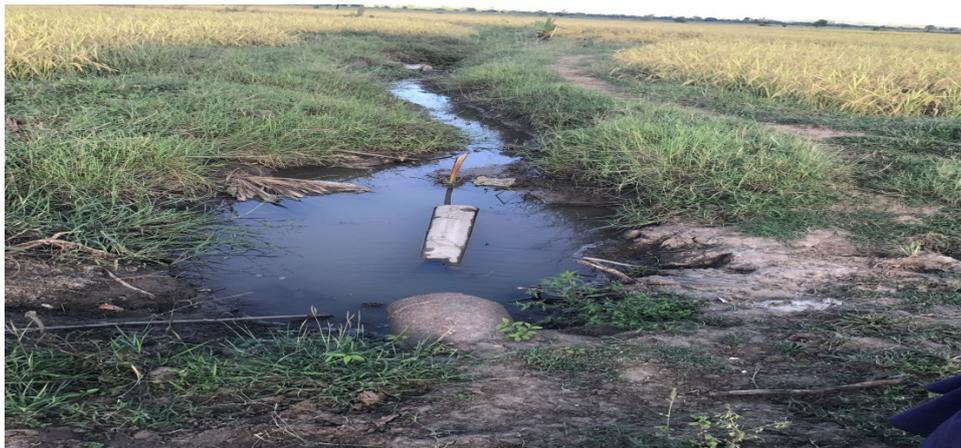
**Figure 4:** Damage of Field-Ditch Canal in the fields of Pae Hlaw Pho Village, Mattaya Township, Saedawgyi Irrigated Area
