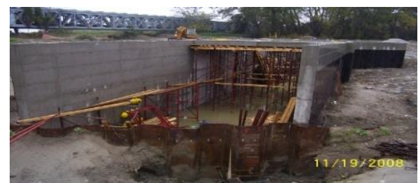
Aqueduct wall construction.
