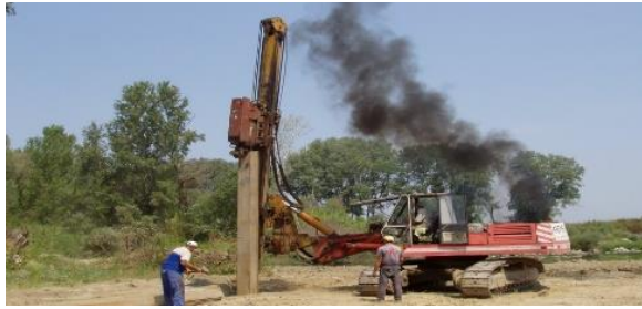
Placement of piles.
