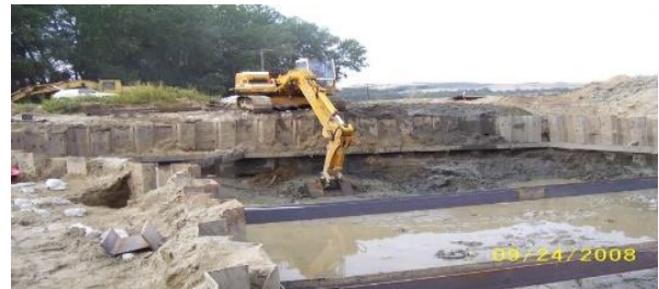
Phase B excavation.
