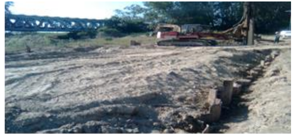
Installed pile series.
