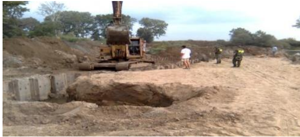
Phase A excavation.
