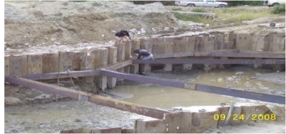
Placement of steel walling – struts.
