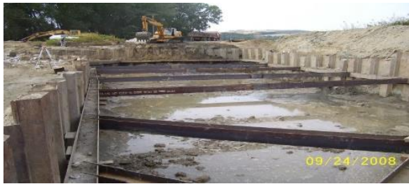
Installed steel walling – struts.
