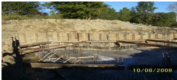
Aqueduct floor construction.
