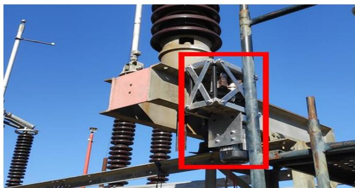
**Figure 5:** Vibrator positioned in the disconnect
